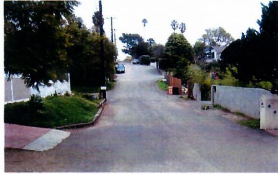
Calle Cita Challenge: Low point in roadway
