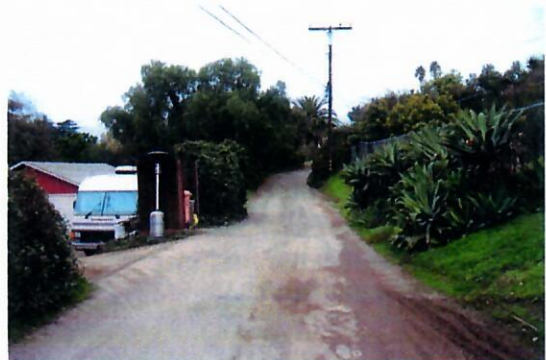
Vista Vallejo – Looking North Challenge: Narrow road
